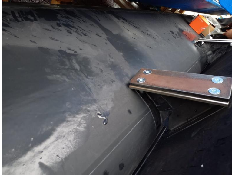
Figure 1: Installing plates over the lashing points
